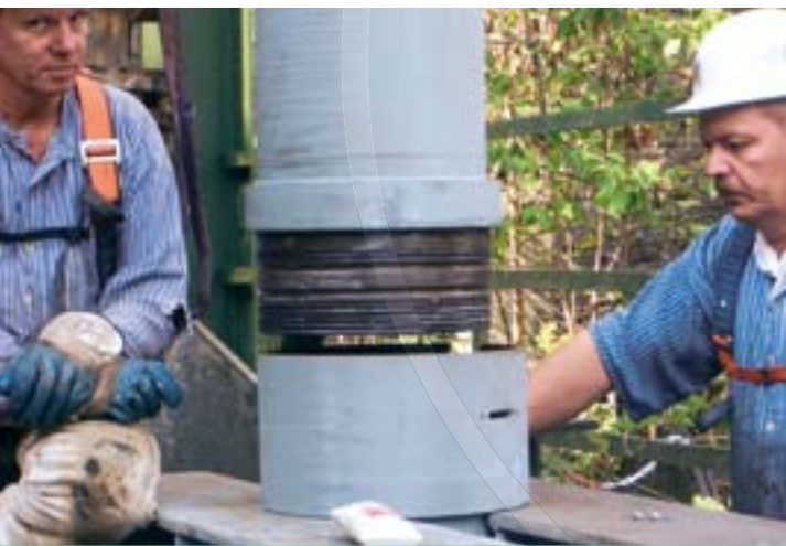
Installation of a ZSM Pipeline
