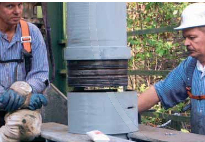
Installation of a ZSM Pipeline
