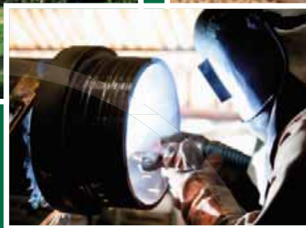
Welding of the spigot end and pipe
